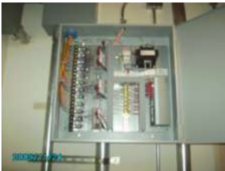
12 circuit simple relay panel tied into existing EMS
